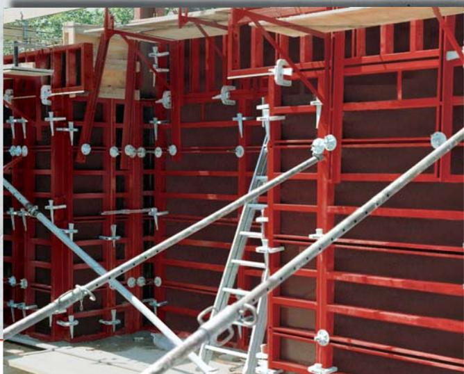
Even large-panel formworks of varying element widths can be used to shutter any ground plan.
