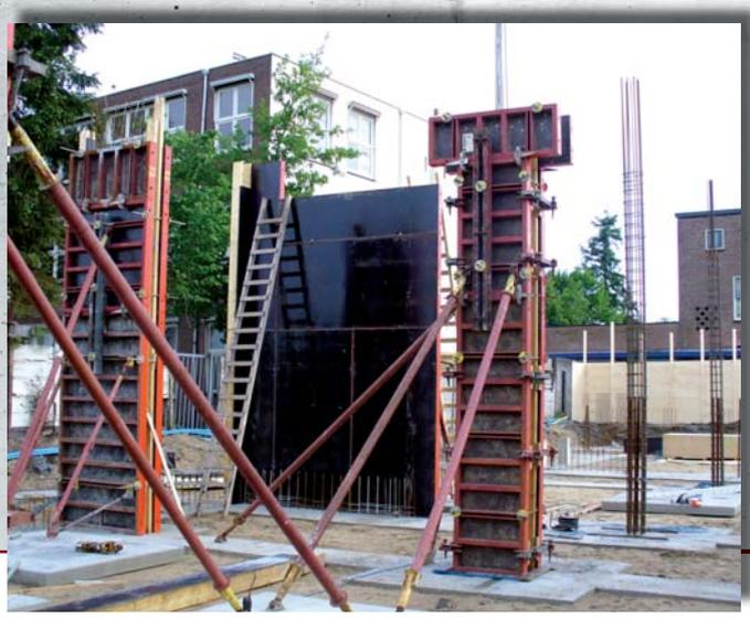
Even complicated ground plans are easy to shutter using just standard elements. Single-faced walls are lined with FEBE shoring frames.
